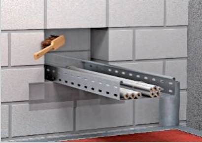
Clean the layer and attach the lining aids, e.g. adhesive tape.
