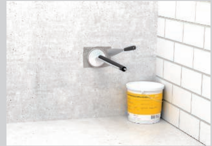
Adjust the foam plugs to installations using a knife and create smoke gas-tight sealing of the sealings using the ASX coating compound.
