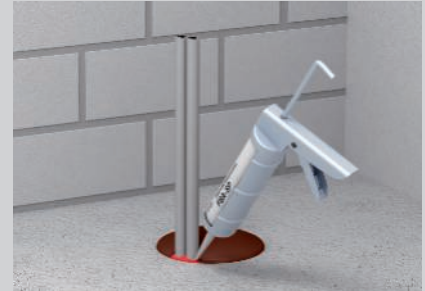
Residual joints are closed off with the filler FBA-SP.
