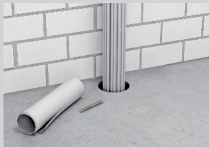
Preparation of the cable insulation.
