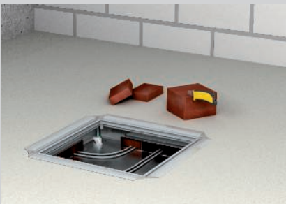
Cut thin strips for the duct compartments.
