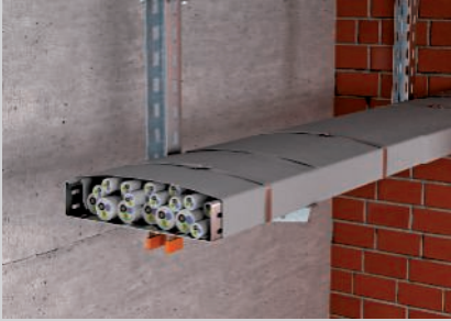
Complete encasement of the suspended cable run.
