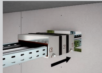
Inserting the box into the wall opening
