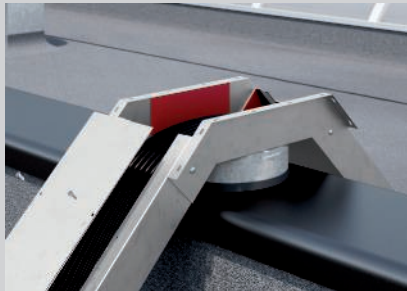
Mounting of the duct cover after cable routing.
