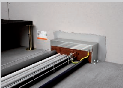
Attaching the equipotential bonding and the identification plate
