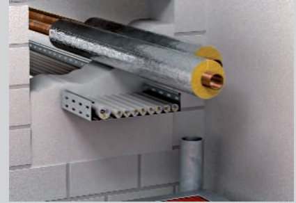
Use approved section insulation for metal pipes.
