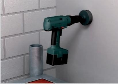
Drilling of a hole with a drill crown.
