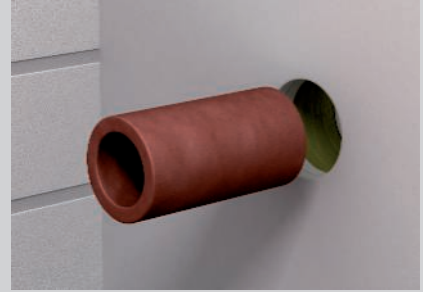
Insertion of the pipe shell in the light-duty partition.
