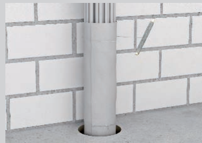
Fixing of the bandage using winding wire.
