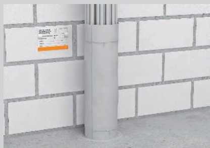
Using mortar, close off the residual insulation opening and mount the identification plate.
