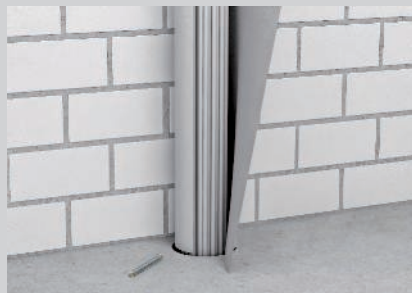
Installation of the fire protection bandage.
